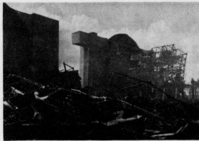
Official U.S. Navy Photo STORM WRECKED BLIMP HANGARS Air Pressure Burst Out Walls
